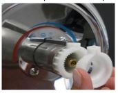
**5**. Using pliers, rotate twisting tool.
