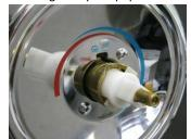
3. Remove cartridge clip \*\*(See Page 2) 4. Place twisting tool on old cartridge.
