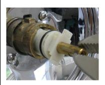
2. Rotate cartridge body 180 degrees and re-install with "H&C" on bottom.
