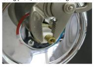
2. Pull stop tube off of valve body.
