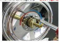
7. Using pliers, pull on cartridge stem.
